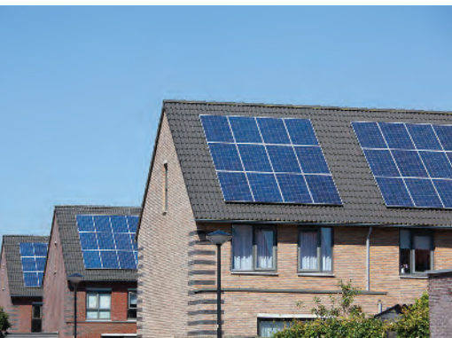
Figure 32.18 These rooftop solar panels are tilted to be face-on to the sun—that is, face-on to the Poynting vector of electromagnetic waves from the sun, so that the panels can absorb the maximum amount of wave energy.
