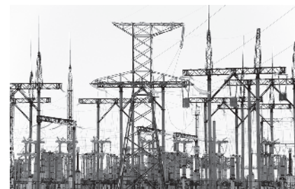
Figure 31.21 Transformer substation where the high-voltage ac (50 kV) in power lines is stepped-down to a lower voltage ac (16 kV).
