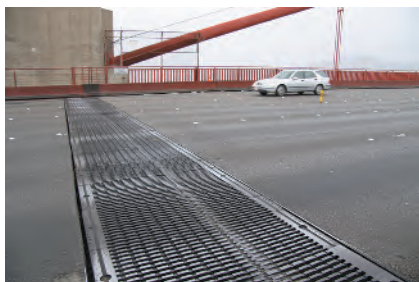
Figure 17.13 Expansion joints on bridges are needed to accommodate changes in length that result from thermal expansion.
